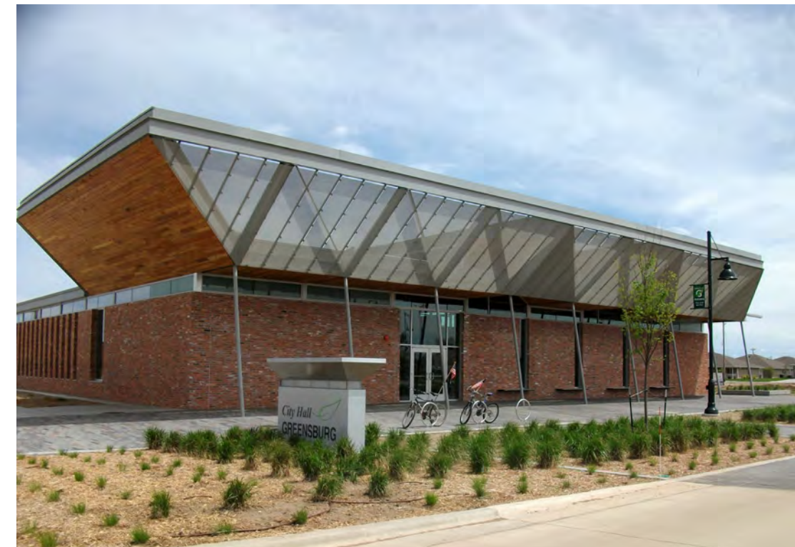
The City Hall building in Greensburg, Kansas, includes solar panels and a ground-source heat pump system that provides heating and cooling.
